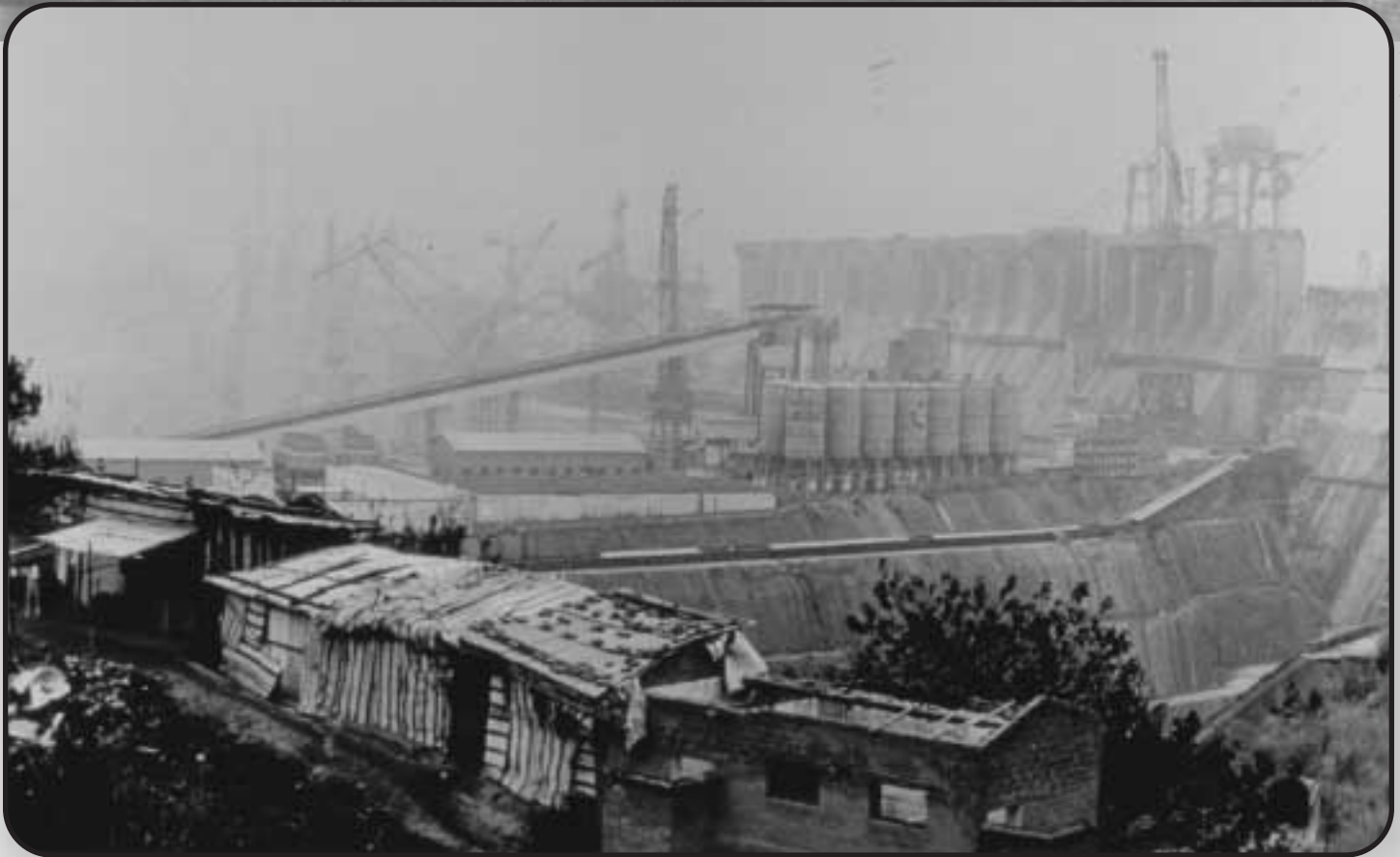
The Three Gorges Dam project. The shanties in the foreground house the construction laborers..
